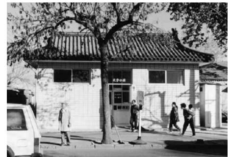
Fig. 8. Public toilet near the Lama Temple, after refurbishment, 5/95. Photo by Tim Geisler.
